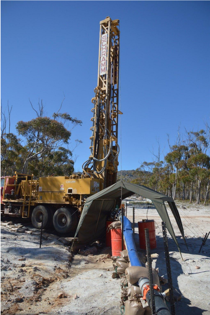
U Deep Aquifer drilling (TMGA)
